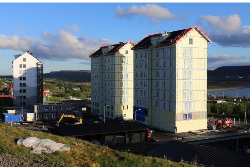
FIGURE A1.39 New residential buildings under construction close to Luossavaara
