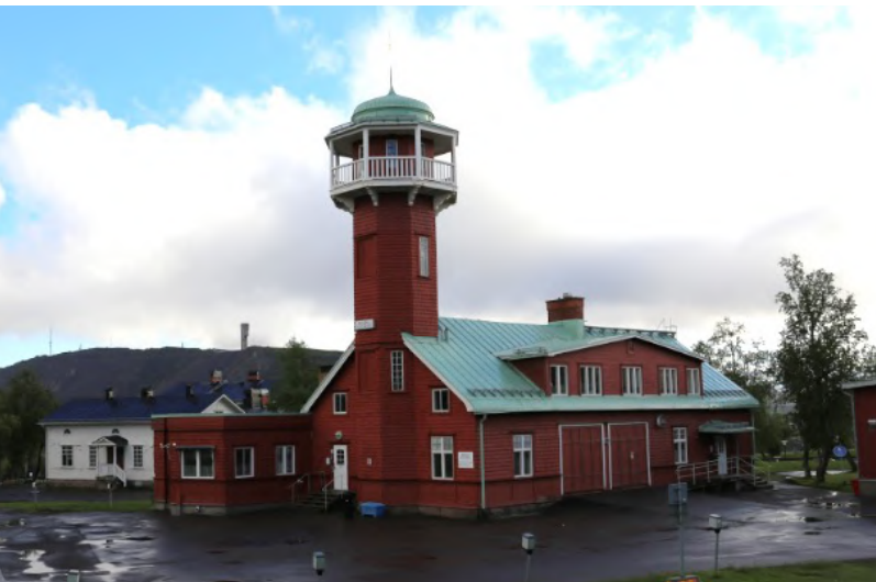
FIGURE A1.31 The old fire station in Kiruna.
