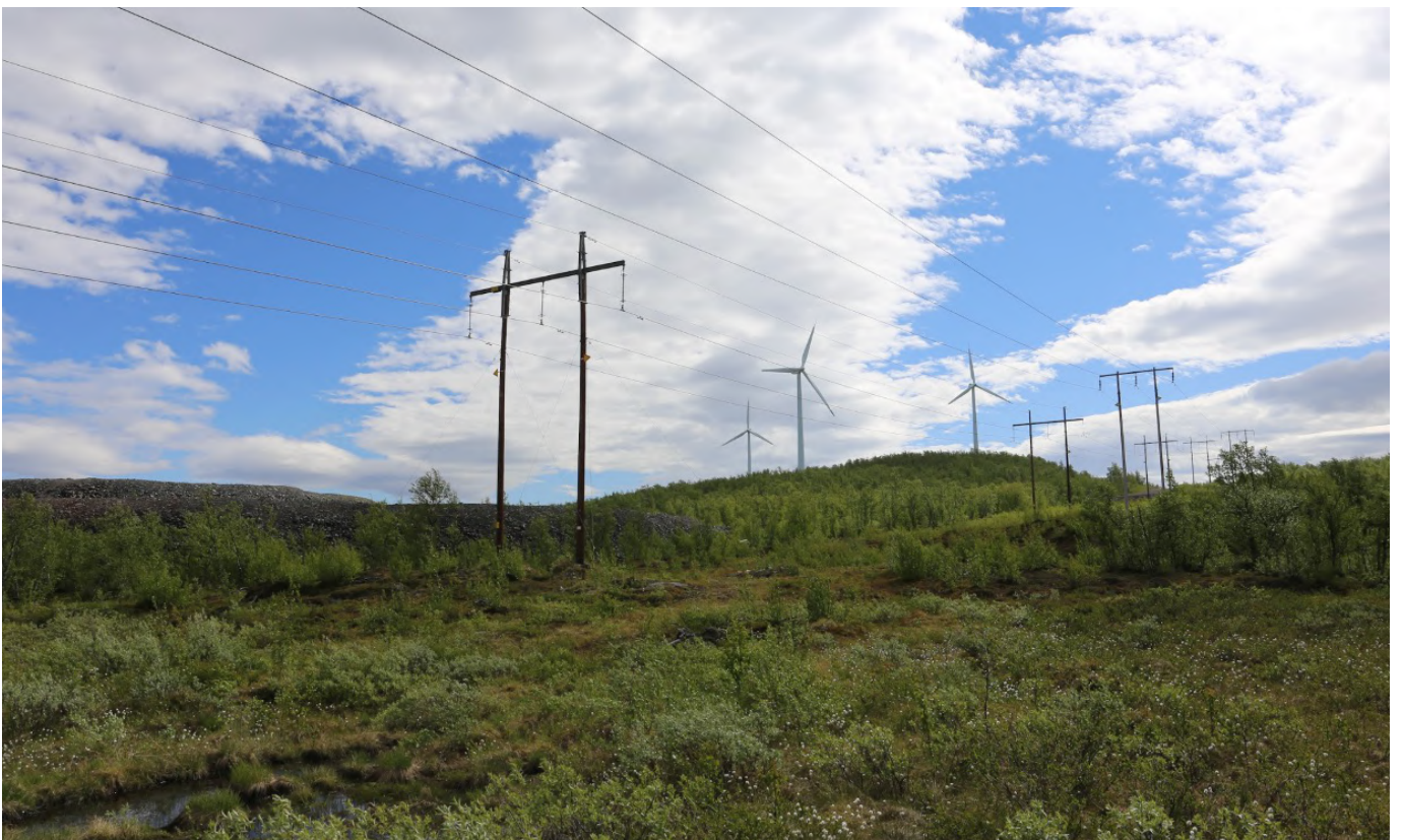
FIGURE A1.7 The high voltage powerlines crossing the north of the site.
