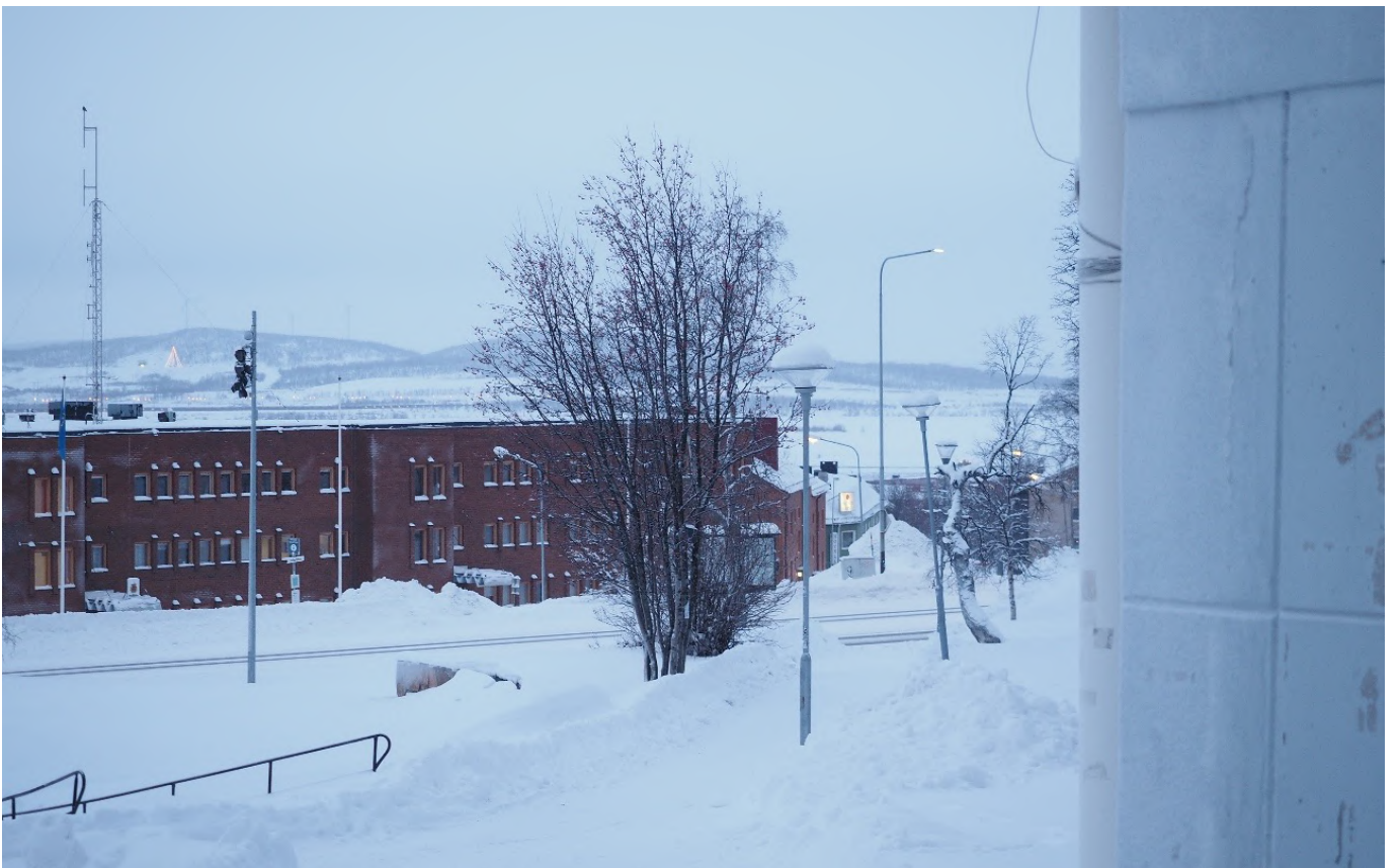
FIGURE 6.11 View of site from the ground in front of the Scandic Ferrum hotel in early December 2021.
